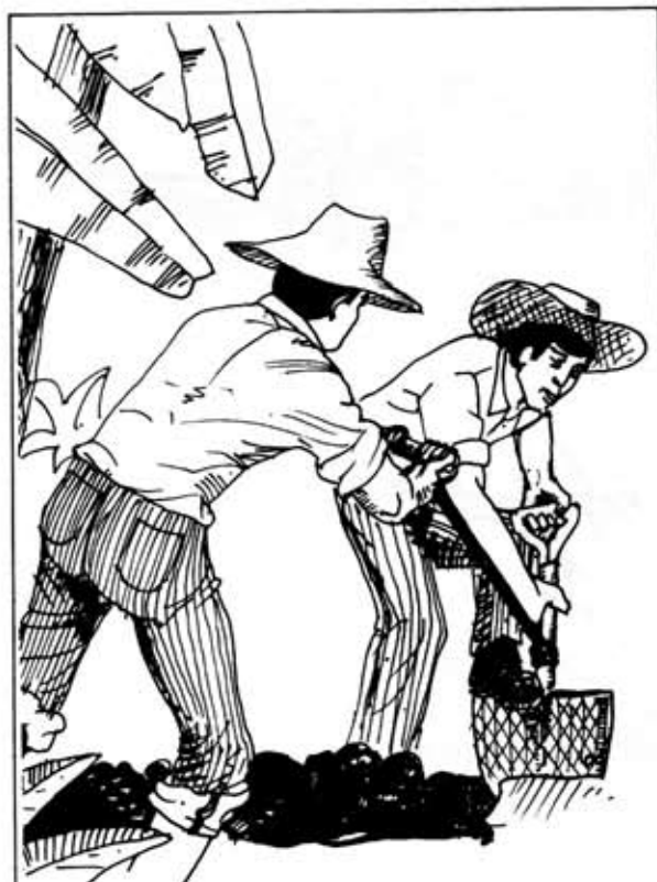
FIGURE 9.26 THE TWO-PERSON SHOVEL A simple, non-tiring digging system for drains, gardens, and terraces.
