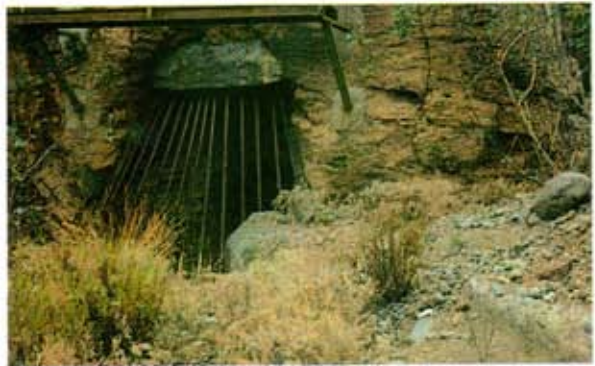
61. LAS PALMAS, CANARY ISLANDS. An arroyo is part-blocked by concrete/stone barrier on right, and bled off via a coarse trash screen to tunnels ( galeria ) and cave storages linked to irrigation systems at lower levels.
