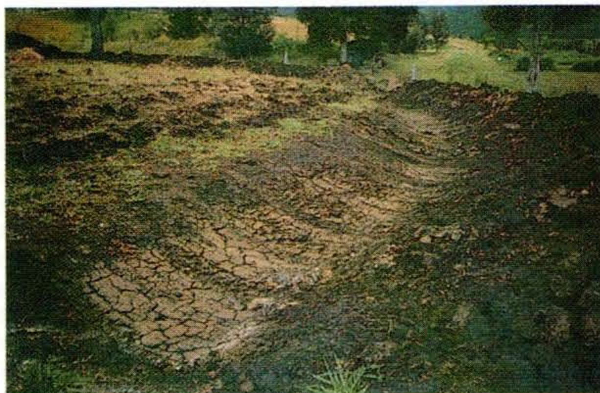
67. PUMPENBIL, NSW, AUSTRALIA. Swale under construction.
