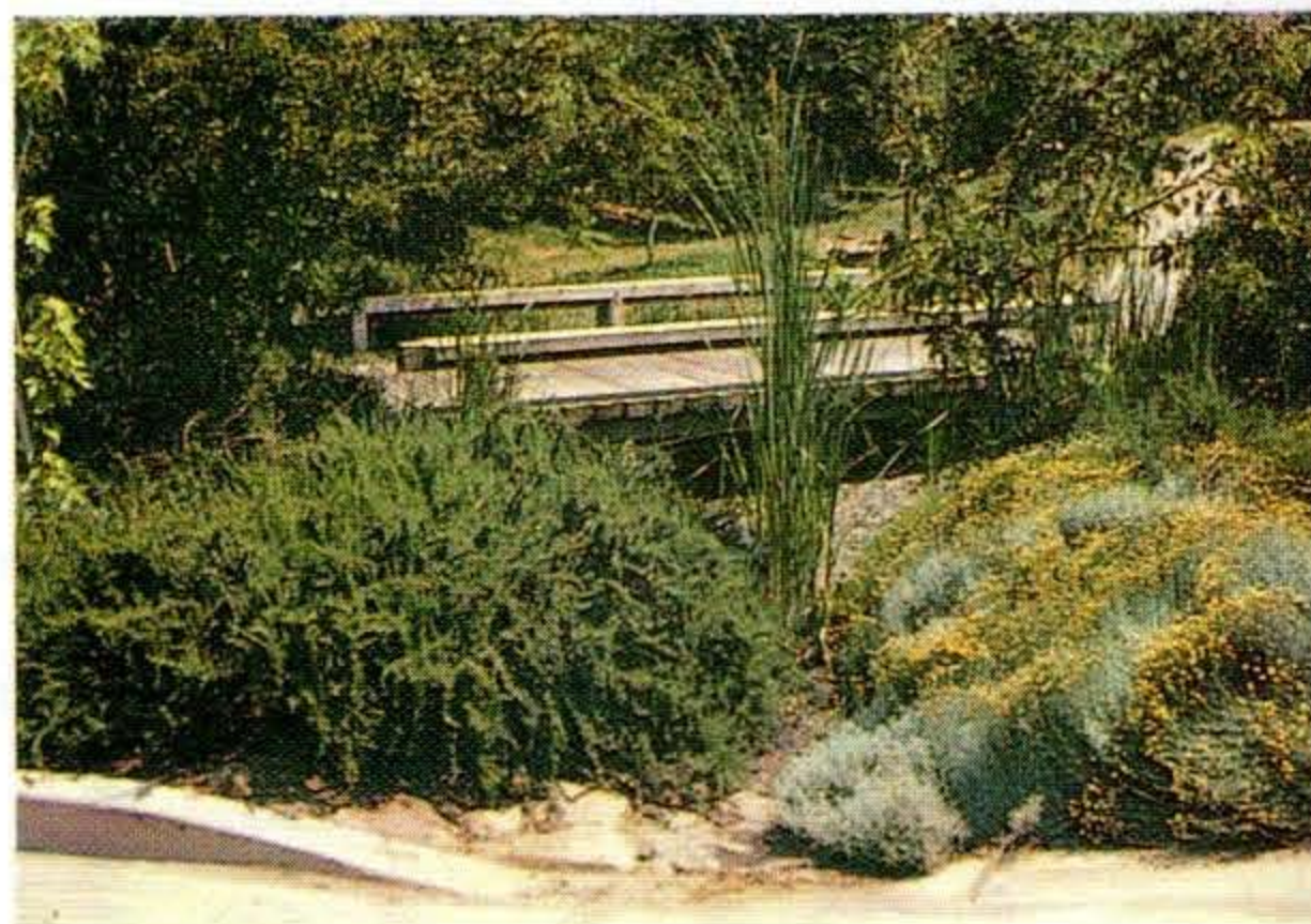
71. VILLAGE HOMES, DAVIS, CA, USA. A gravel-based swale collects water from a suburban road. Because of extensive swaling Village Homes sits on its own deepening, soil-stored, water reservoir in a surrounding desert.
