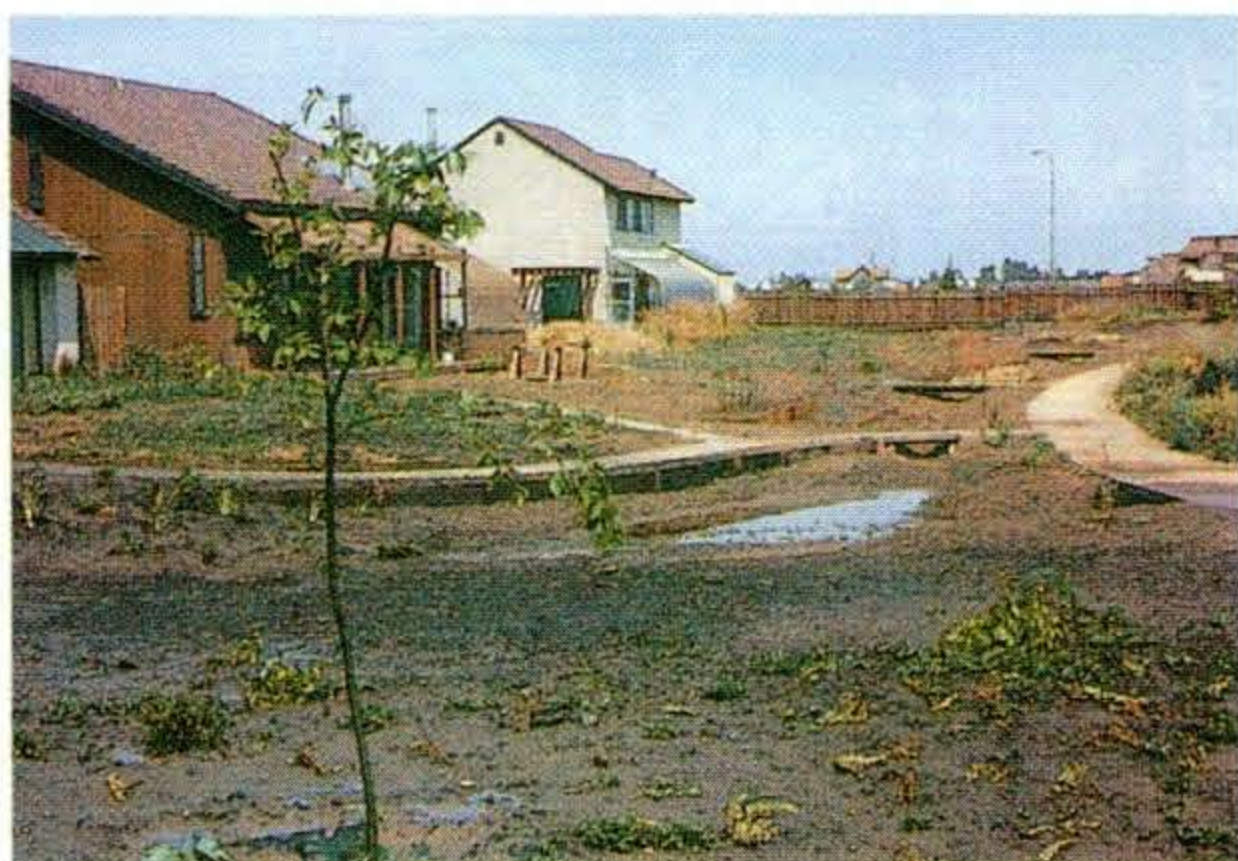
69. VILLAGE HOMES, DAVIS, CA, USA. Michael Corbett, designer/developer. New swale area being planted.
